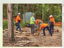
Reinforcement cages being placed in the holes
