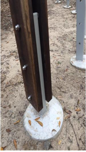
A detail of the spigot/post assembly. Note the carefull detailing of the steel work, the bolt locations and the concrete base. Eventually when the surrounding pathwork and landscaping has been completed the concrete base will no longer be seen.
