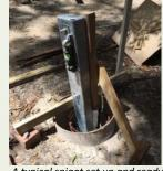
A typical spigot set up and ready for the concrete placement
