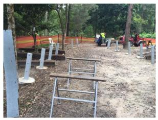
Stirrups all in place, concrete poured and waiting for the timber posts to be installed
