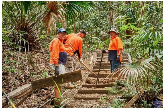
Allan, Ray and Jeff replacing rotten steps
