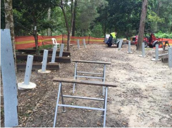
*Stirrups all in place, concrete poured and waiting for the timber posts to be installed*
