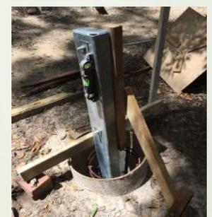
A typical spigot set up and ready for the concrete placement
