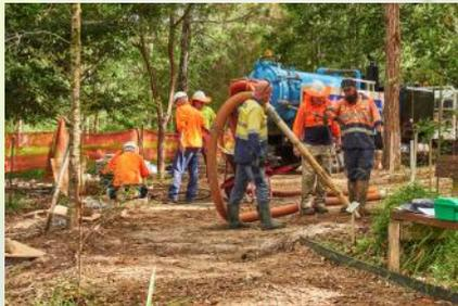
The pier holes were excavated by a vacuum/suction method in order to minimise damage to principal tree roots...a high pressure water jet displaces the soil and a giant vacuum cleaner sucks it up...the process whilst very impressive took a lot longer than we anticipated...
