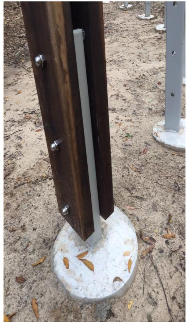
*A detail of the spigot/post assembly. Note the careful detailing of the steel work, the bolt locations and the concrete base. Eventually when the surrounding pathwork and landscaping has been completed the concrete base will no longer be seen.*
